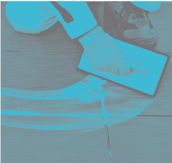
**1** Installation must be carried out using normal adhesives for porcelain stoneware or specific, high-performance adhesives depending on the size or particular applications.
