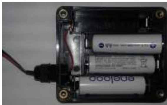
Fig 17 – Replacing battery in battery box
