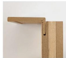
Plywood sandwich panel frame on hinge side
